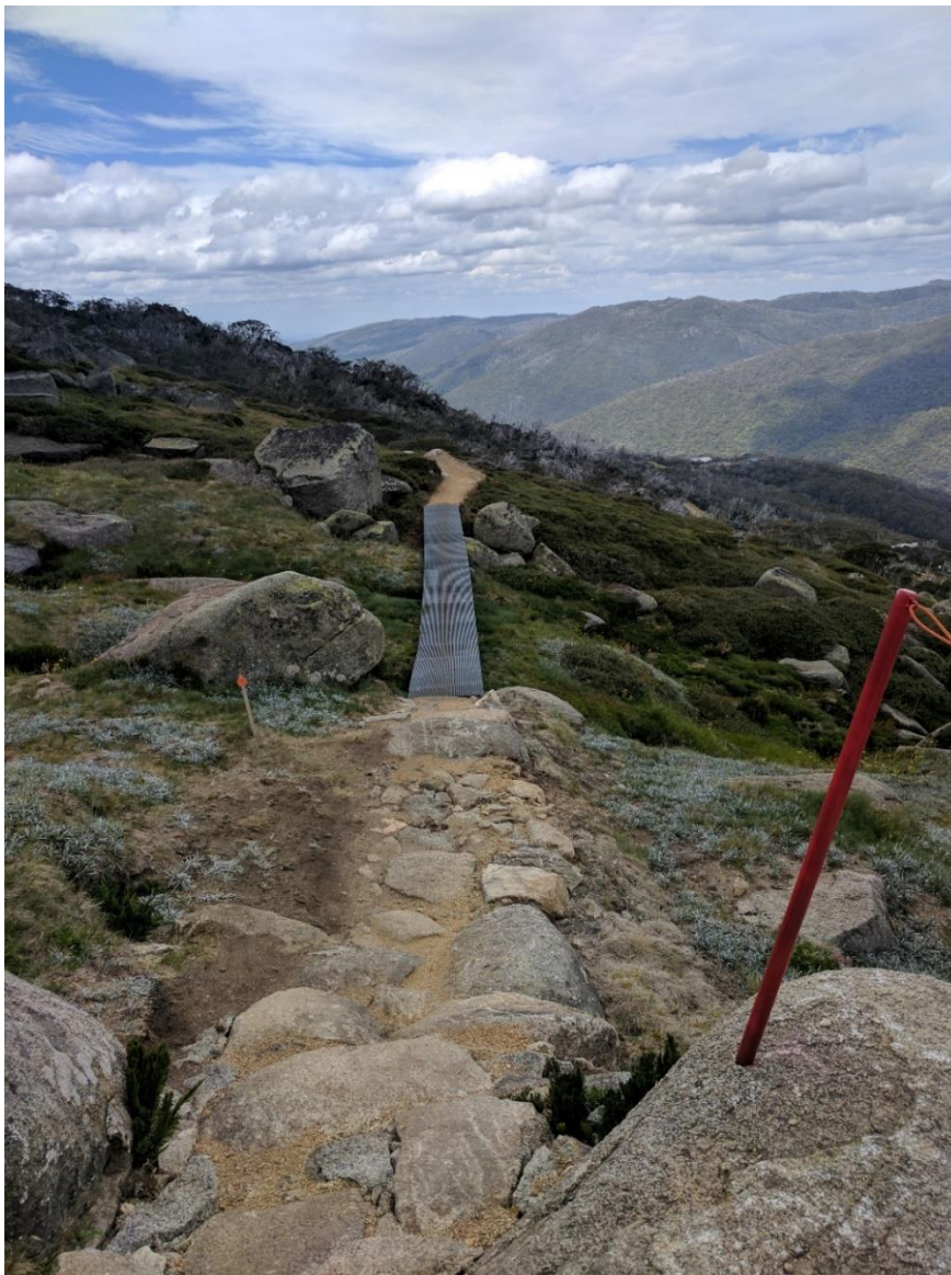
Figure 36: Example of rock armouring on the All-Mountain Trail
