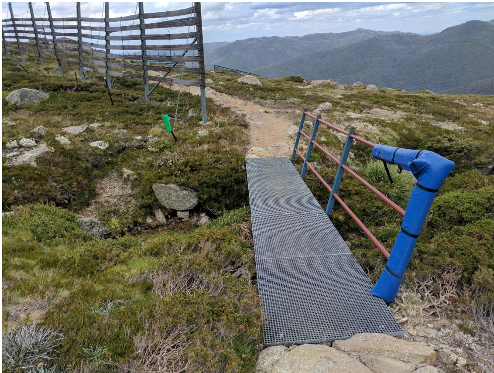
Figure 38: Platform with a guard rail on the All-Mountain Trail
