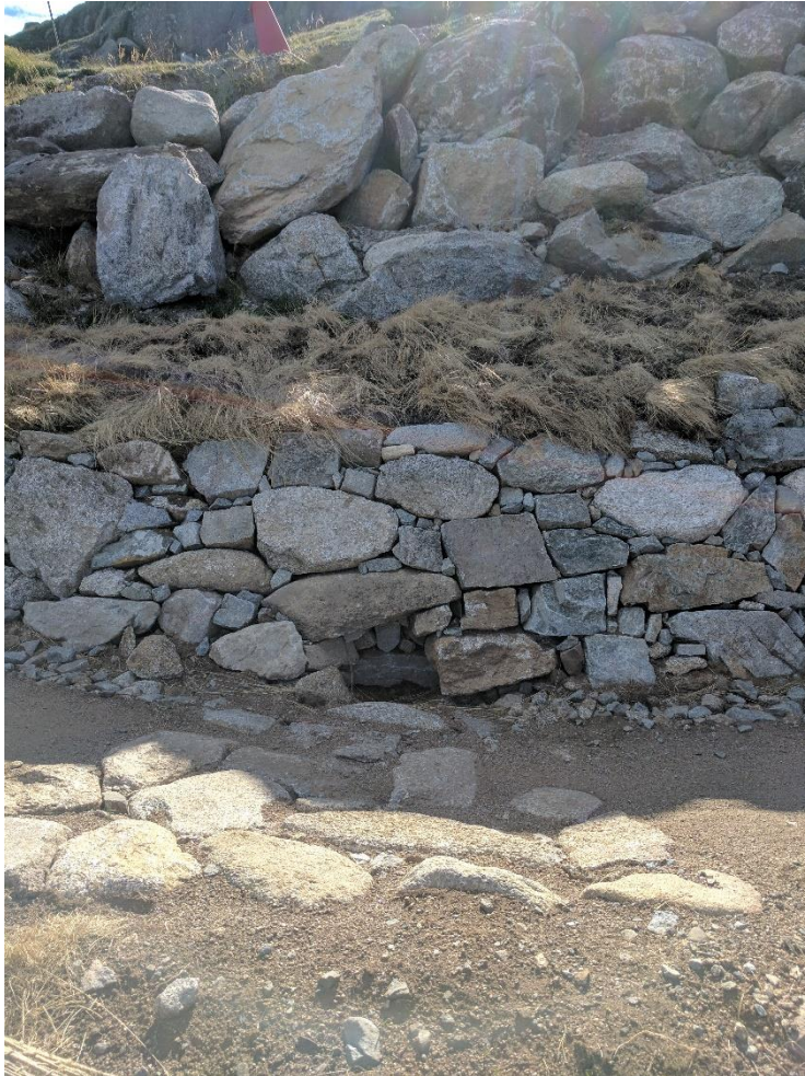
Figure 34: Example of a drain dip, rock hardened on the All-Mountain Trail
