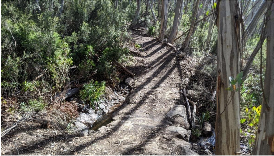
Figure 35: Example of rock armouring on the Lower N4 Trail
